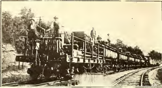
SPRINKLING TRAIN FOR EXTENSIVE APPLICATION OF WEED KILLER
